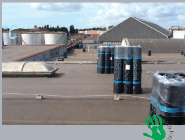
**PROJECT SPECIFICATIONS:** polyolefin polymer APP compound suitable for exposed multilayer systems with self-protected finish, painted or under heavy protection; finishing element in multi-layer systems and for waterproofing projects used with bituminous waterproofing membranes of the Enduring Quality range.
